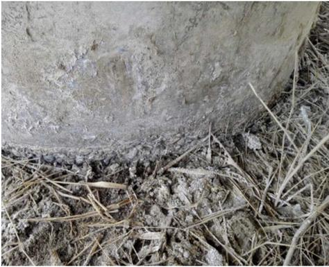
Fig. 4. Pier concrete wet and dry cycle erosion damage situation
